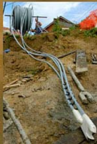
5 vertical geothermal probes going 100m underground
