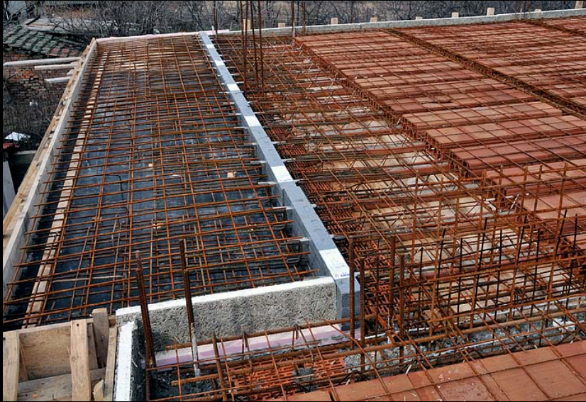
Load bearing thermal break for balconies
