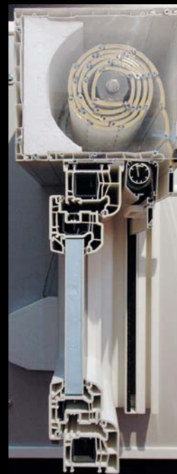
Insulated shutter, low-e glazing, argon fill
