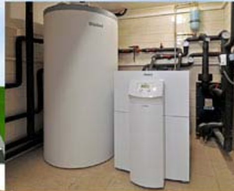
Vaillant GeoTHERM VWS 300/2 geothermal heat pump and storage buffer
