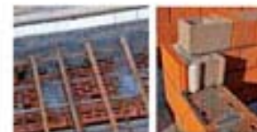
Figure XV.vi - Placing horizontal and vertical coverage elements with thermal insulation on Apartment house Amadeo (photo Kace Beodan, www.beodan.com)
