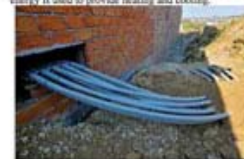
Figure XV.vii - Passage of the geothermal probes into Amadeo building (photo Kace Beodan)
