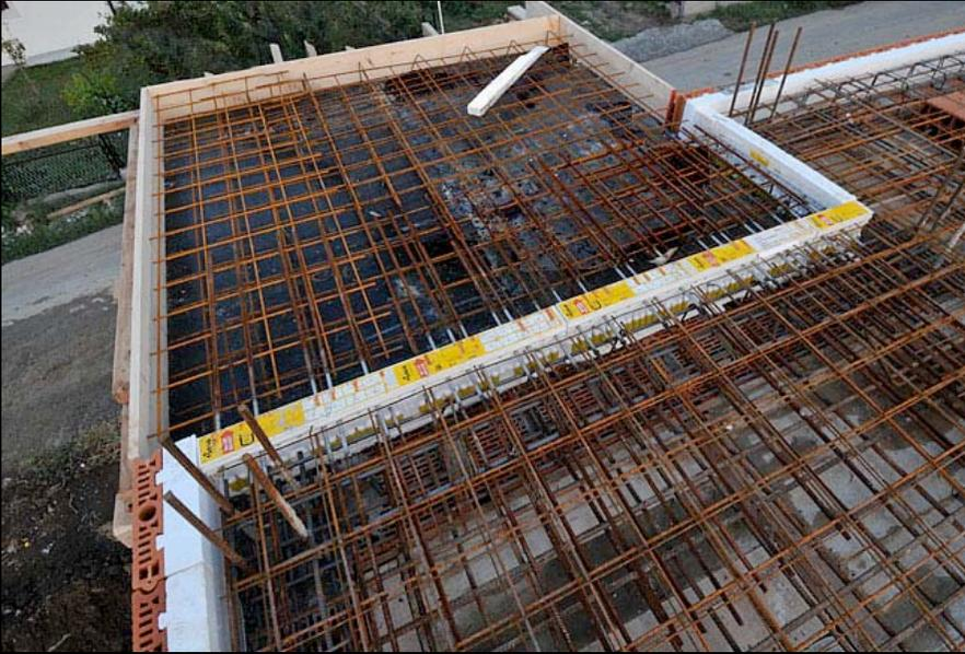
Schoeck Isokorb: load bearing thermal break for balcony
