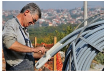
Priprema i montiranje Raugeo sonde za spuštanje u bušotinu. Preparing and assembling Raugeo probe for the installation in the borehole.
