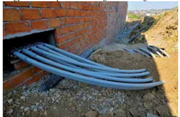
Figure XV.vii - Passage of the geothermal probes into Amadeo building (photo Kuće Beodom)
